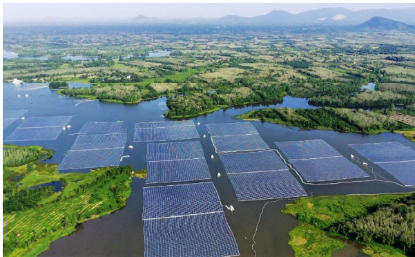
Floating Solar at Tasik Danau Tok Uban, Kelantan
